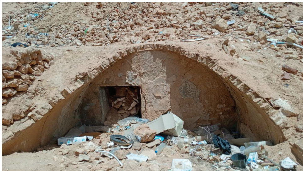
Fig22.2. The ruins of the Hammam in Hamma
